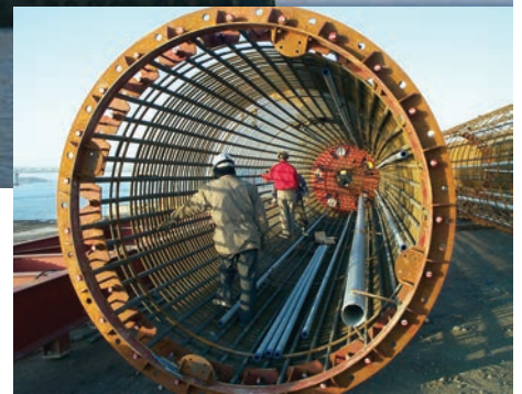
Reinforcing cage for the O-cell test site in Korea
