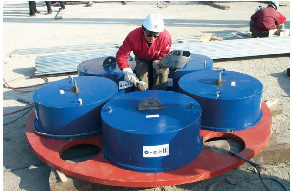
Workers checking O-cells at the Incheon bridge site
